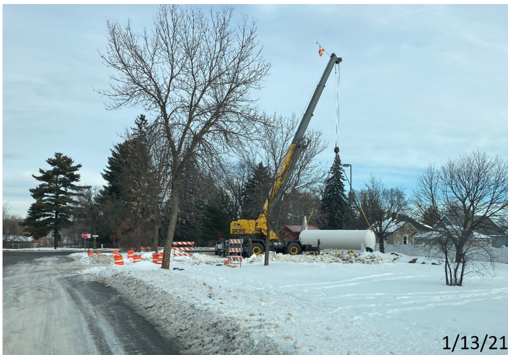
LOX tank delivery and installation
