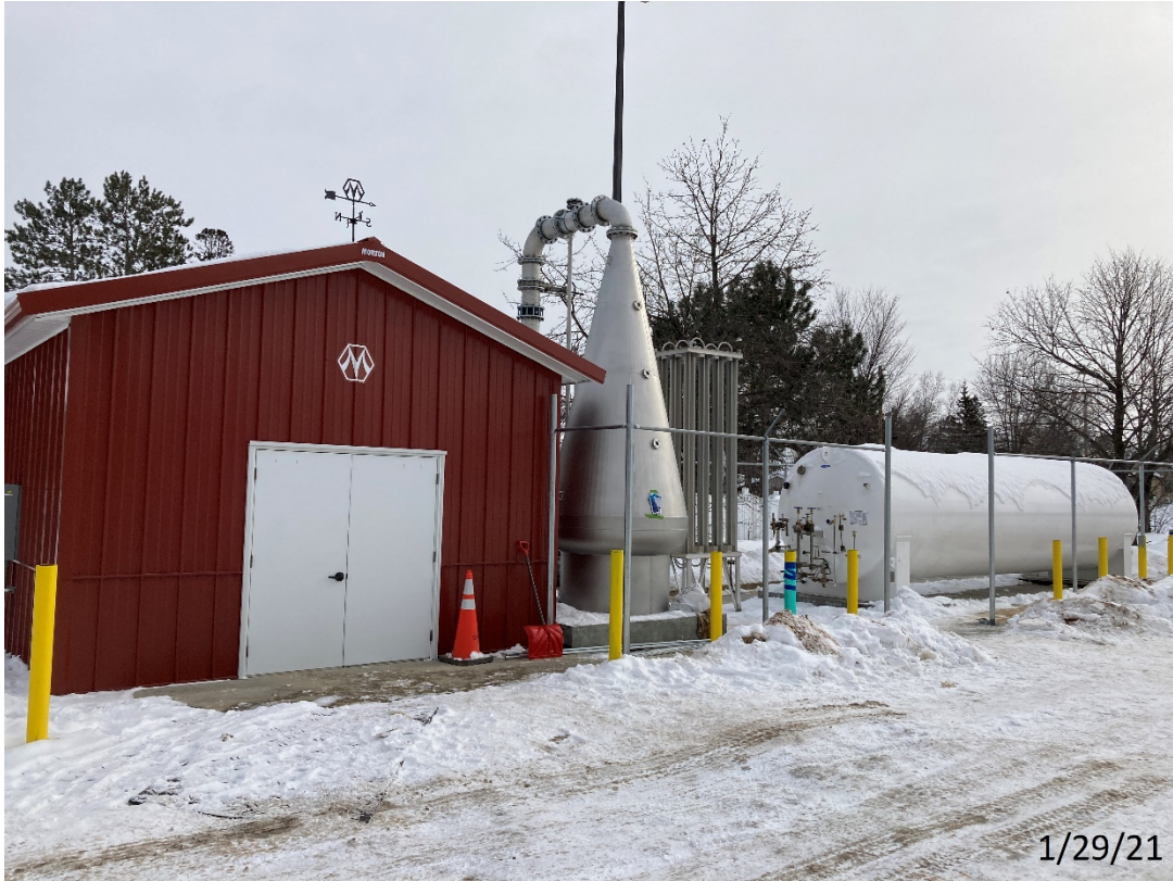
Inlet piping to the cone set in place (joint GRPUC effort).
